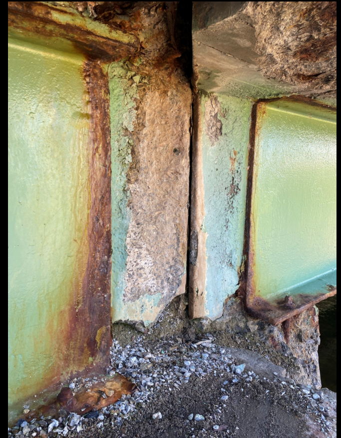
Concrete pier condition
