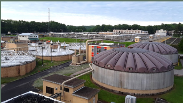
Monroe County Water Resource Recovery Facility
