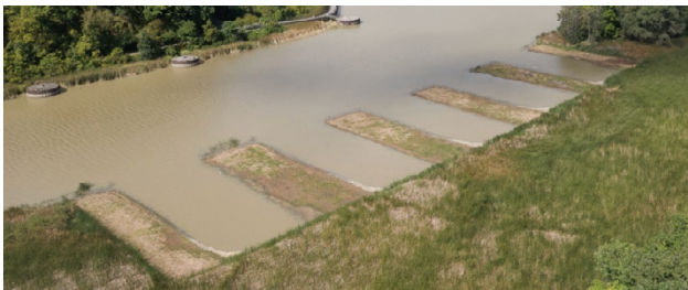
Figure 9: Completed Wetland C North site
